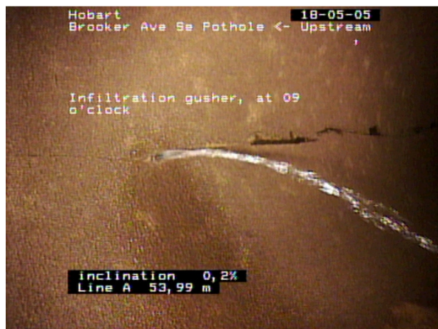
Figure 1: Infiltration leak
